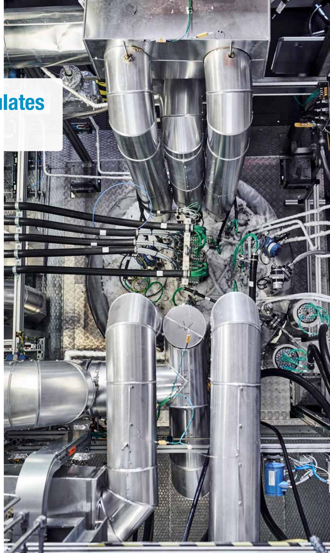
Water moderates, slows down fast neutrons and hampers the splitting of minor actinides. "Transmutation cannot occur in these circumstances", explains Katrien. In the MYRRHA design, a eutectic alloy of lead (44.50%) and bismuth (55.50%) will cool the core without slowing down the fast neutrons. "The coolant flows through the reactor core, absorbs heat, rises and sheds this heat in the heat exchangers before dropping back down into the core. This cools the core."
